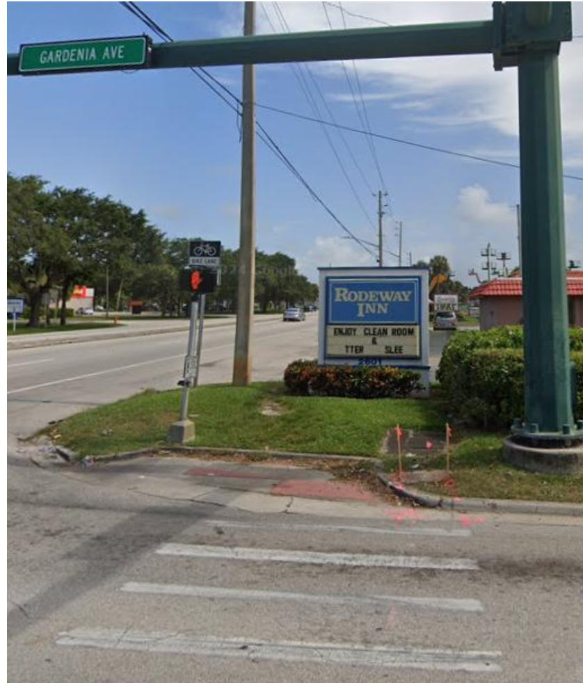
Sidewalk Gap/Non-ADA Compliant Pedestrian Ramp
