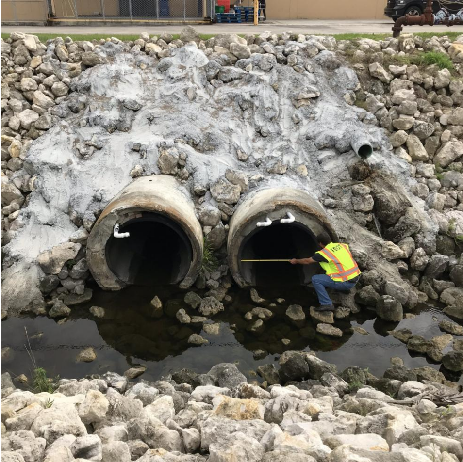
Lined Pipes at Mayflower Canal
